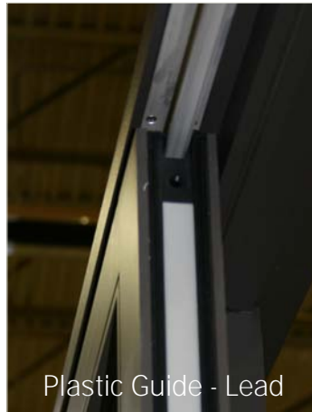
On a slight angle slide the top of the door over the track
